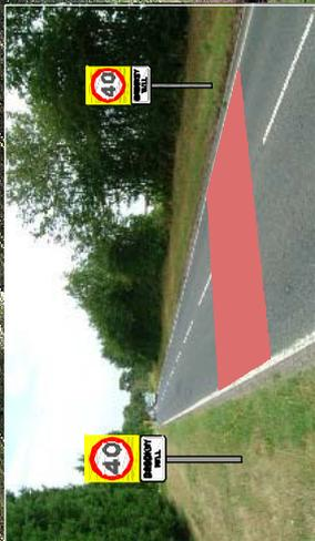
Proposed 'gateway' feature to highlight the entry into the existing 30mph speed limit on Wheldrake Lane
